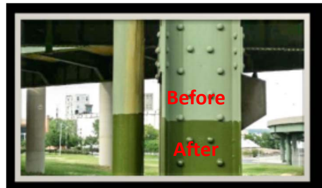
Lewis & Clark Viaduct - Kansas City, MO
